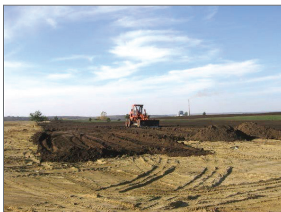
Figure 2. Topsoil placement upon preparation for agriculture reclamation in „Drmno“ mine
